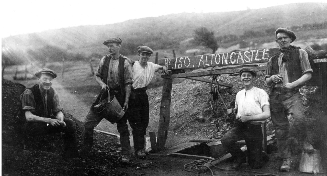
Adit mining, Alton Castle, near Cheadle | 1920
