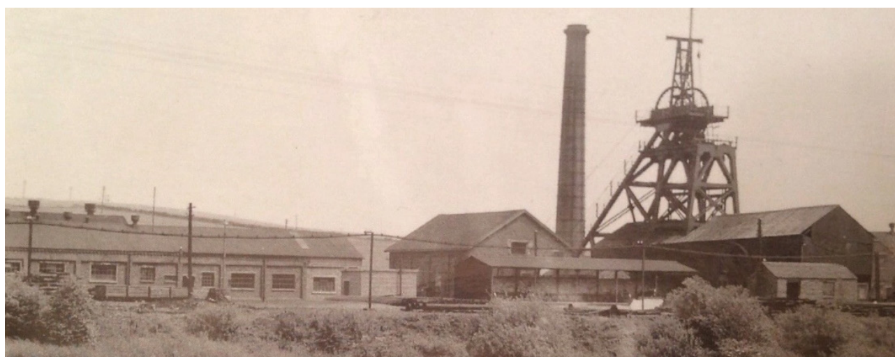
Kents Lane Pit, Silverdale, Newcastle under Lyme
